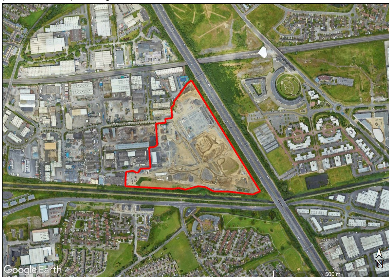
Figure 1.1. Aerial view showing the Echelon Clondalkin DC Services Limited facility (outlined in red) in the greater context.
