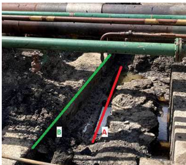
Figure B. Services Beneath the HFO Spill – Middle Trench
