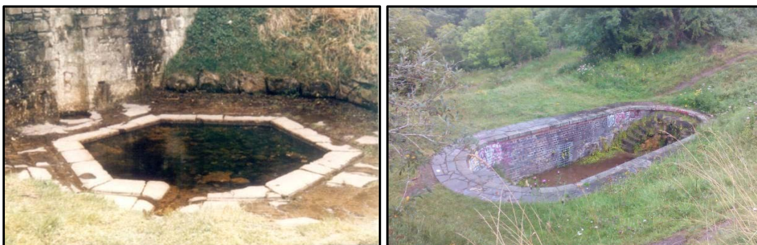
Photographs 1 & 2: Spa well (c. 1983, GSI) showing original well, hexagonal cistern and overflow, and outdoor Roman-style bath (24 th August 2016)
