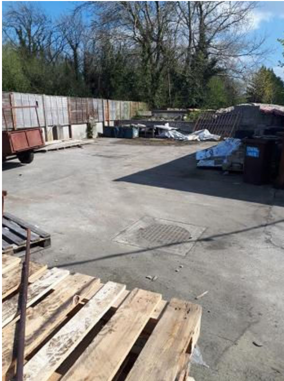
Photo 1: Yard area currently designated for Firewater Retention
