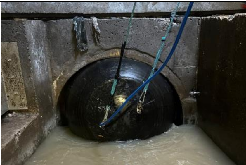
Inflatable flow stopper in place
