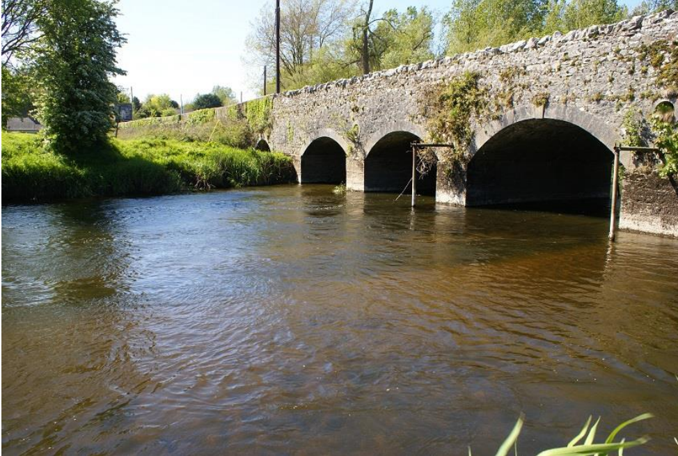
Site 1. Tallyho Bridge
