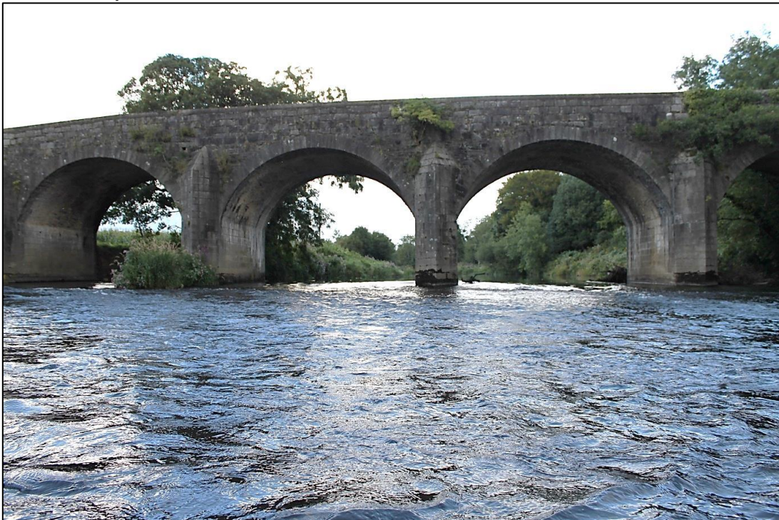
Figure 3.11: Monitoring Point 11 (New Bridge)
