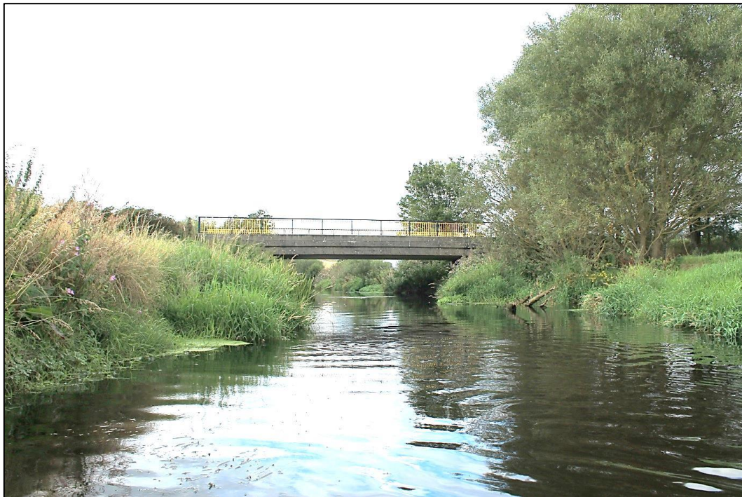
Figure 3.9: Monitoring Point 9 (Balisland Bridge)
