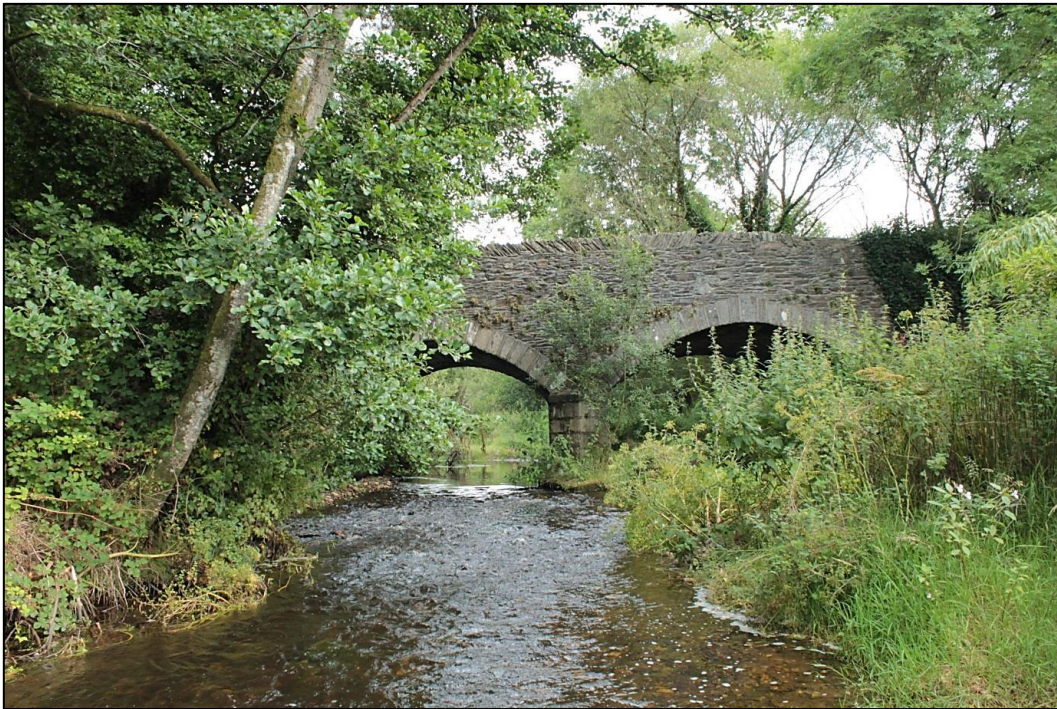
Figure 3.1: Monitoring Point 1 (Greenhall Bridge)
