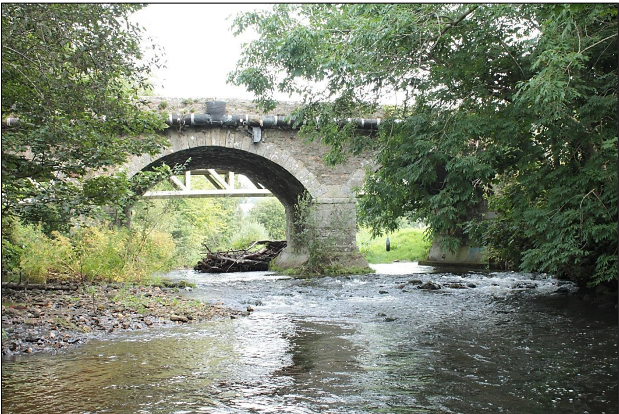
Figure 3.3: Monitoring Point 3 (Shillelagh Bridge)
