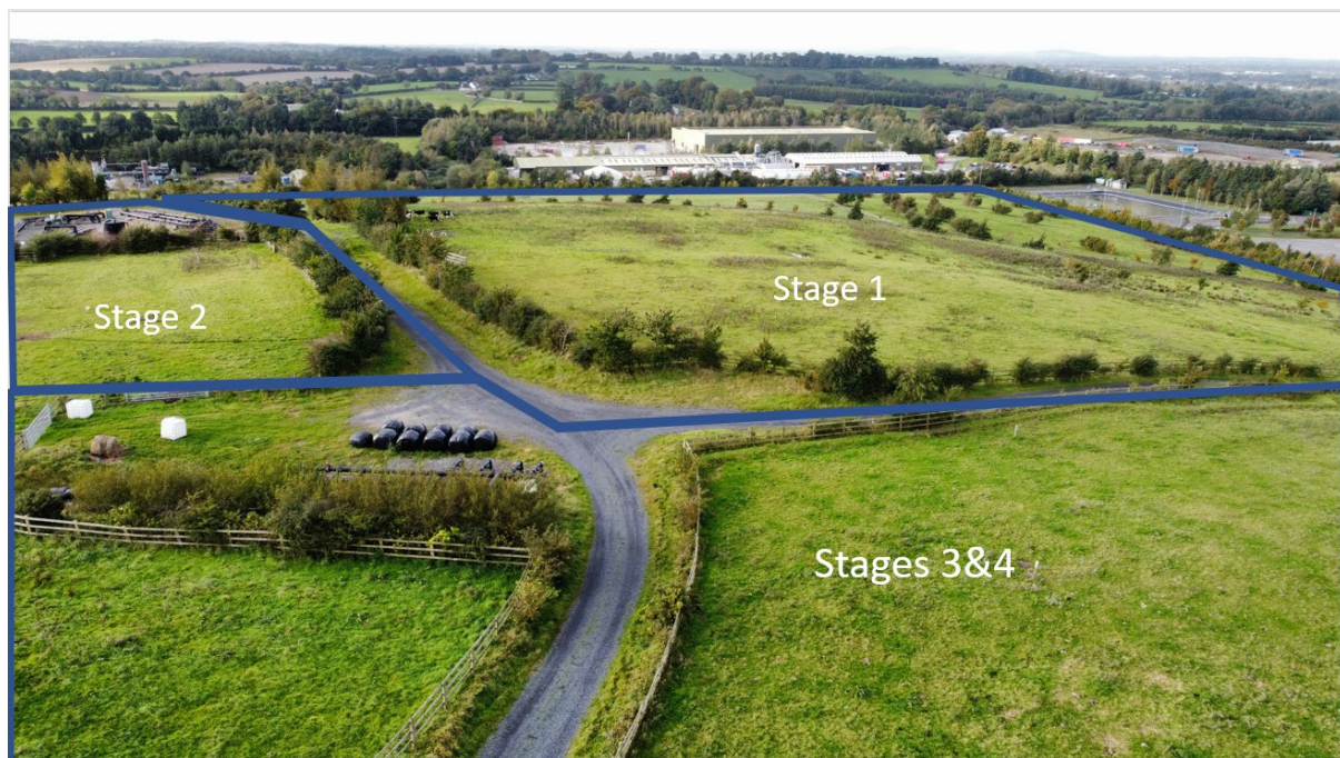
Figure 3: Aerial view from East to West – towards Stage 1 of the Site
