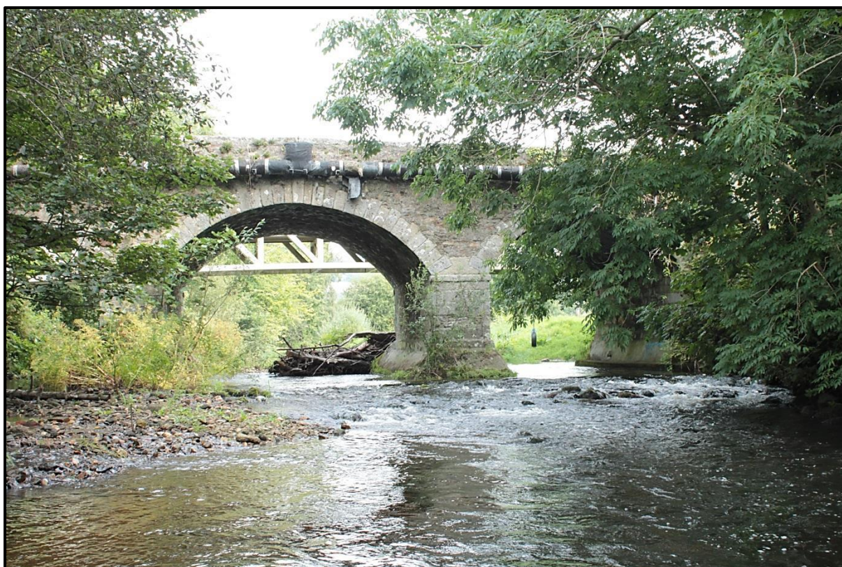
Figure 3.3: Monitoring Point 3 (Shillelagh Bridge)
