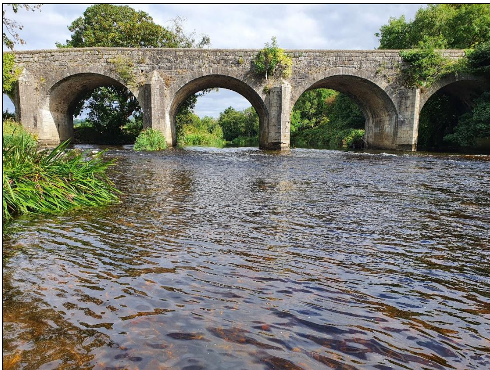
Figure 3.11: Monitoring Point 11 (New Bridge)
