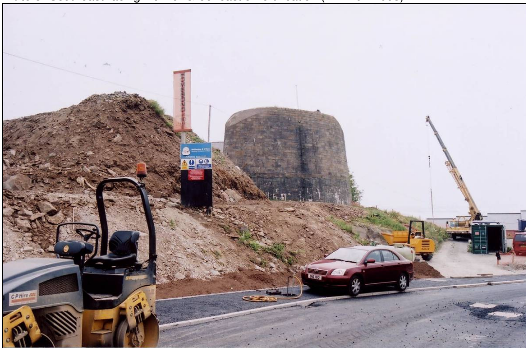
Plate 4: Southeast-facing view of Martello Tower located adjacent to Greencastle fortification.
