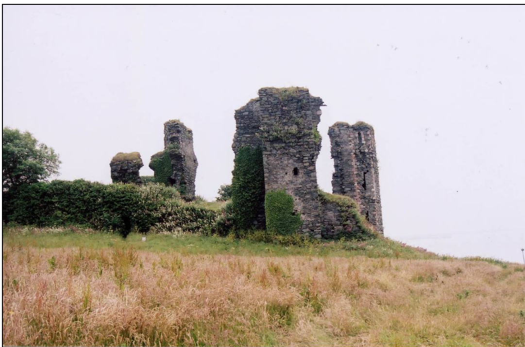
Plate 3: Southeast-facing view of Greencastle Fortification (RMP:022-003).
