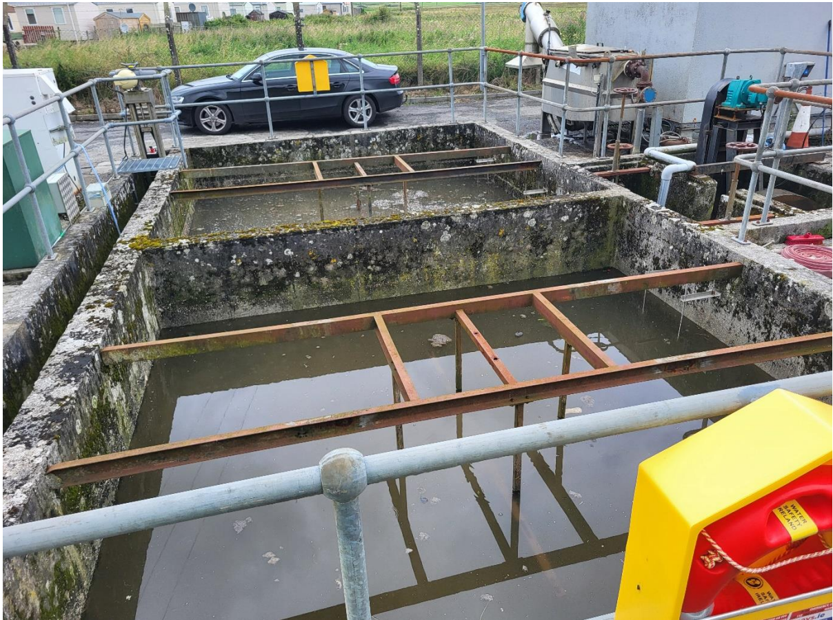
Photograph No. 3: Final clarifiers at the Lahinch WWTP which were found to be flooded due to the plant not discharging during high tides on the day off this site visit (22 nd of July 2025).
