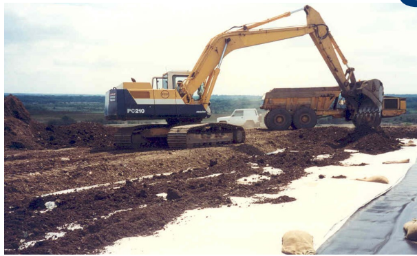
Fig. 13: Placing cover soil
