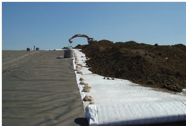
Fig. 6: Pozidrain placed on steep slope
