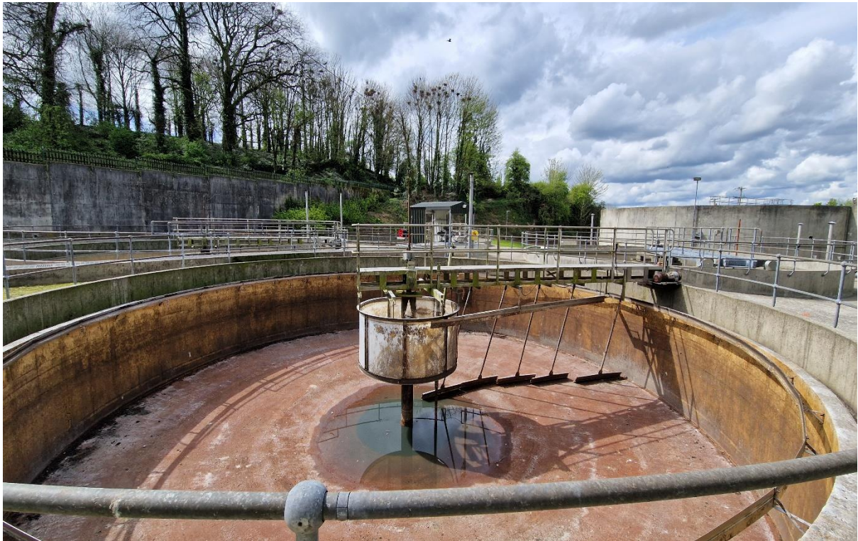
Photograph No. 1: Primary settlement tank not in operation as a result of a breakdown.
