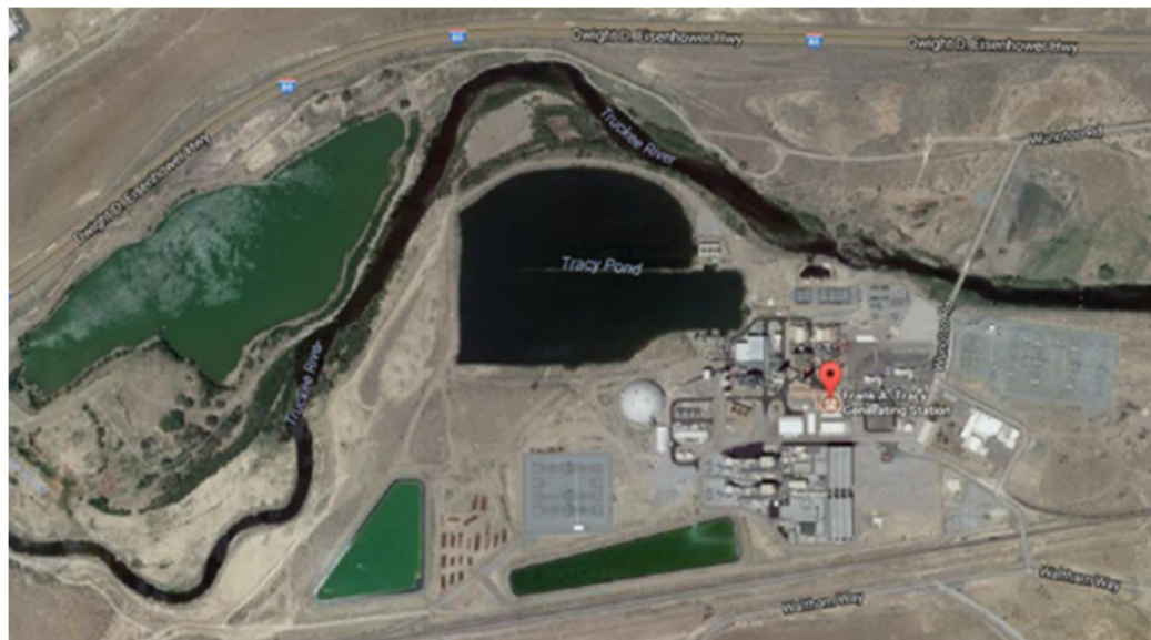
Figure 3-19: Example Cooling Ponds Taking up Large Areas of Land
