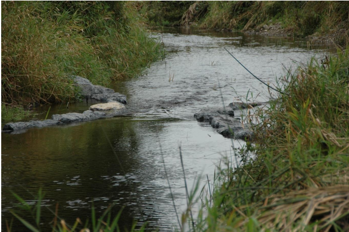
Figure 2 Paired Deflectors under Construction
