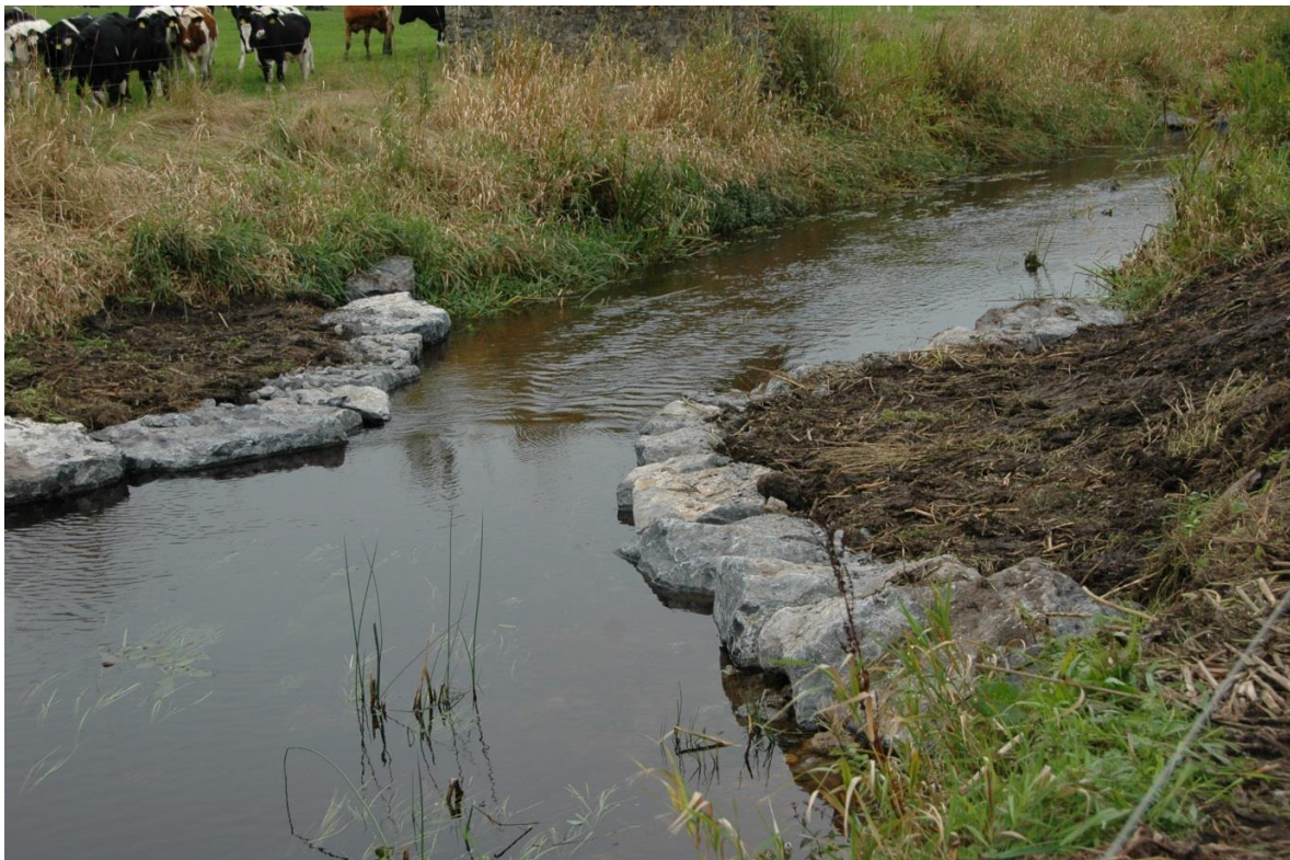
Figure 3 Completed Paired Deflectors, note backfill which will vegetate
