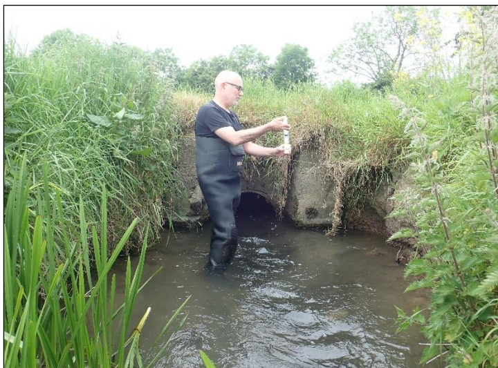
Plate 7 Irish Cement trade effluent outfall to the River Nanny. The outfall stream was visibly cleaner than the receiving water.
