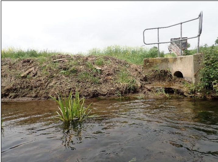
Plate 22 Bank maintenance works on the River Nanny upstream of Site N6.
