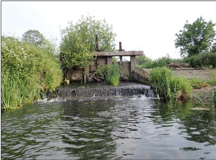
Plate 4 Weir upstream of Site N1 ponds water and also reduces the flow at Site N1.
