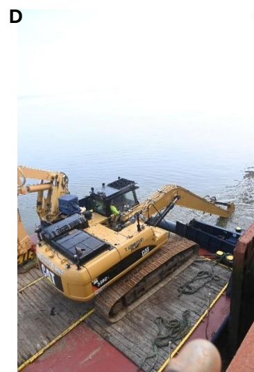
Figure 3. Ploughing operations at the Aughinish Alumina marine terminal jetty. (A) the bed levelling unit is raised here, this is used for ploughing operations, (B) the Fastnet Sound carrying out ploughing operations, the bed levelling unit is dropped to the sea bed (C) & (D) excavating operations being conducted from the Fastnet Sound by the long arm tracking machine.
