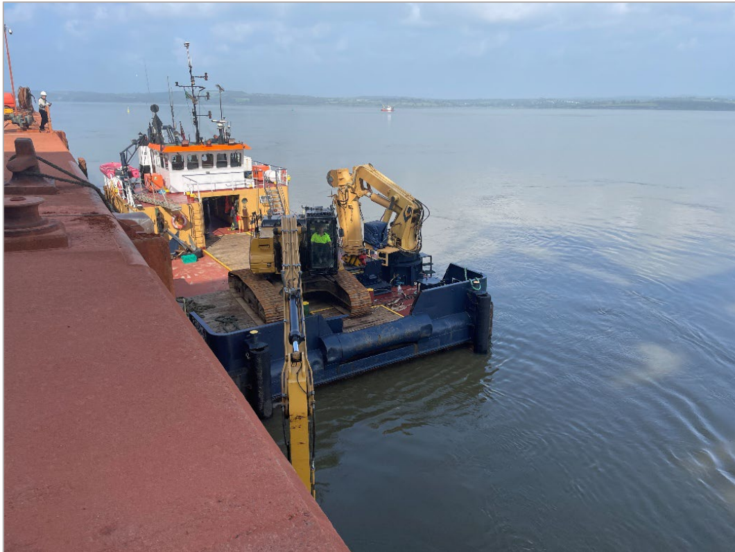
Plate 1: Area A machine dredging
