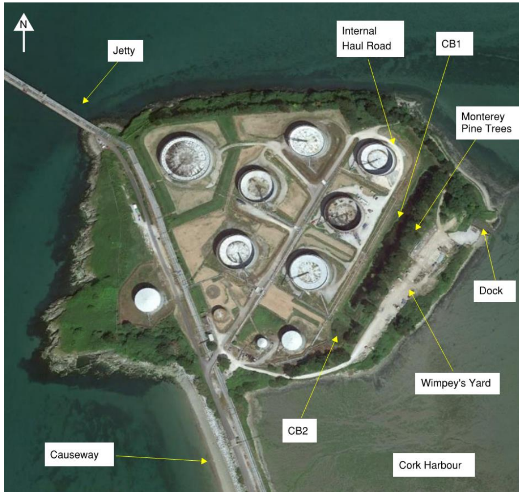
Figure 2: Overview of existing site
