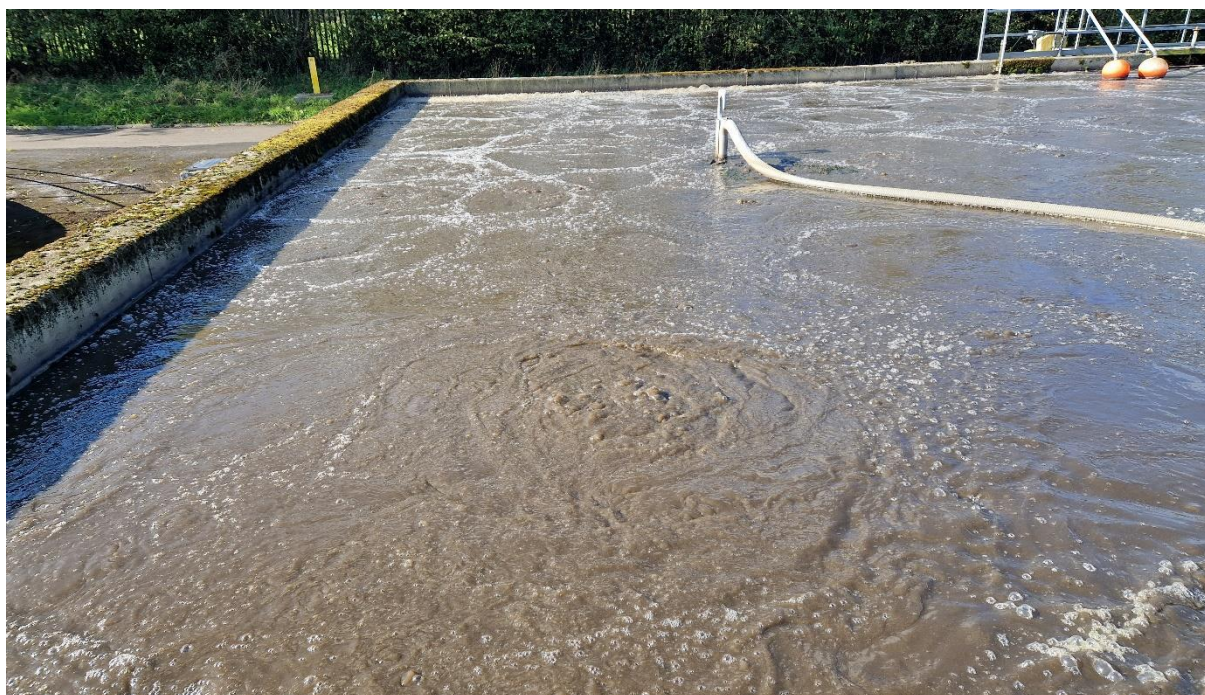
Photograph No. 1: A corner of the aeration tank that did not appear to be oxygenated.
