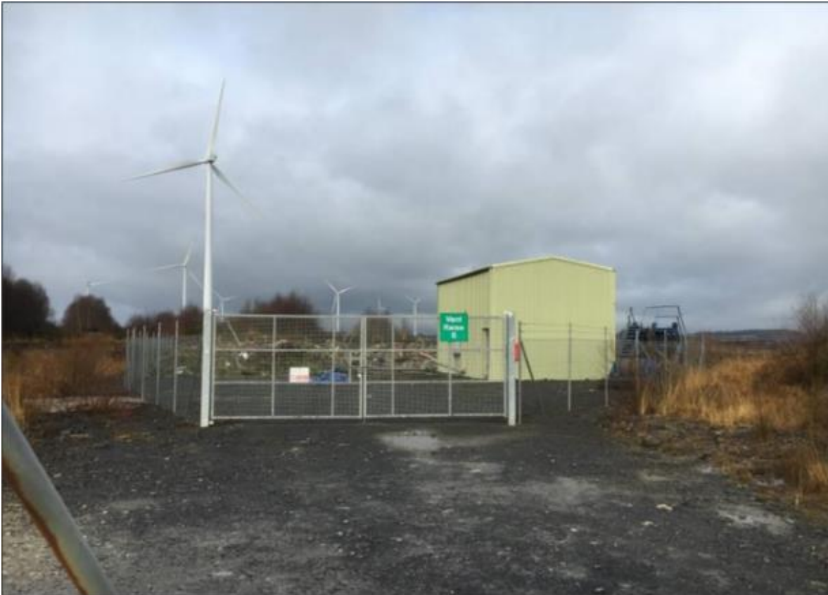
Figure 3-5: Ventilation Shaft 6 pre demolition
