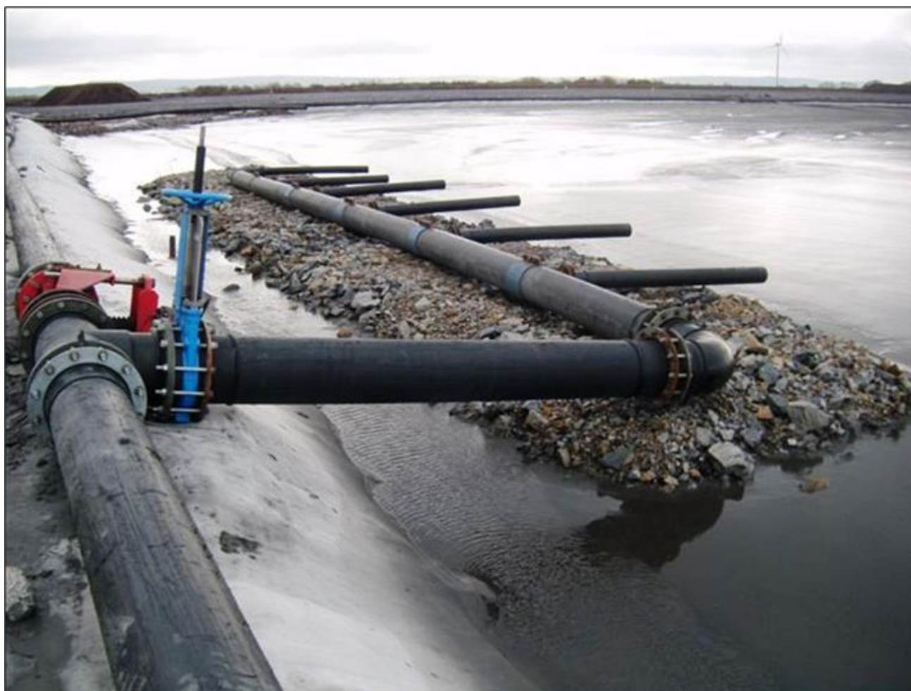
Figure 4-5: Spigot pipe system
