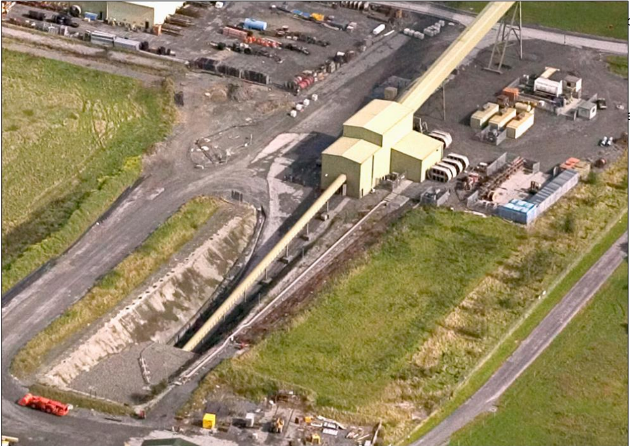
Figure 3-10: Mine Portal pre demolition
