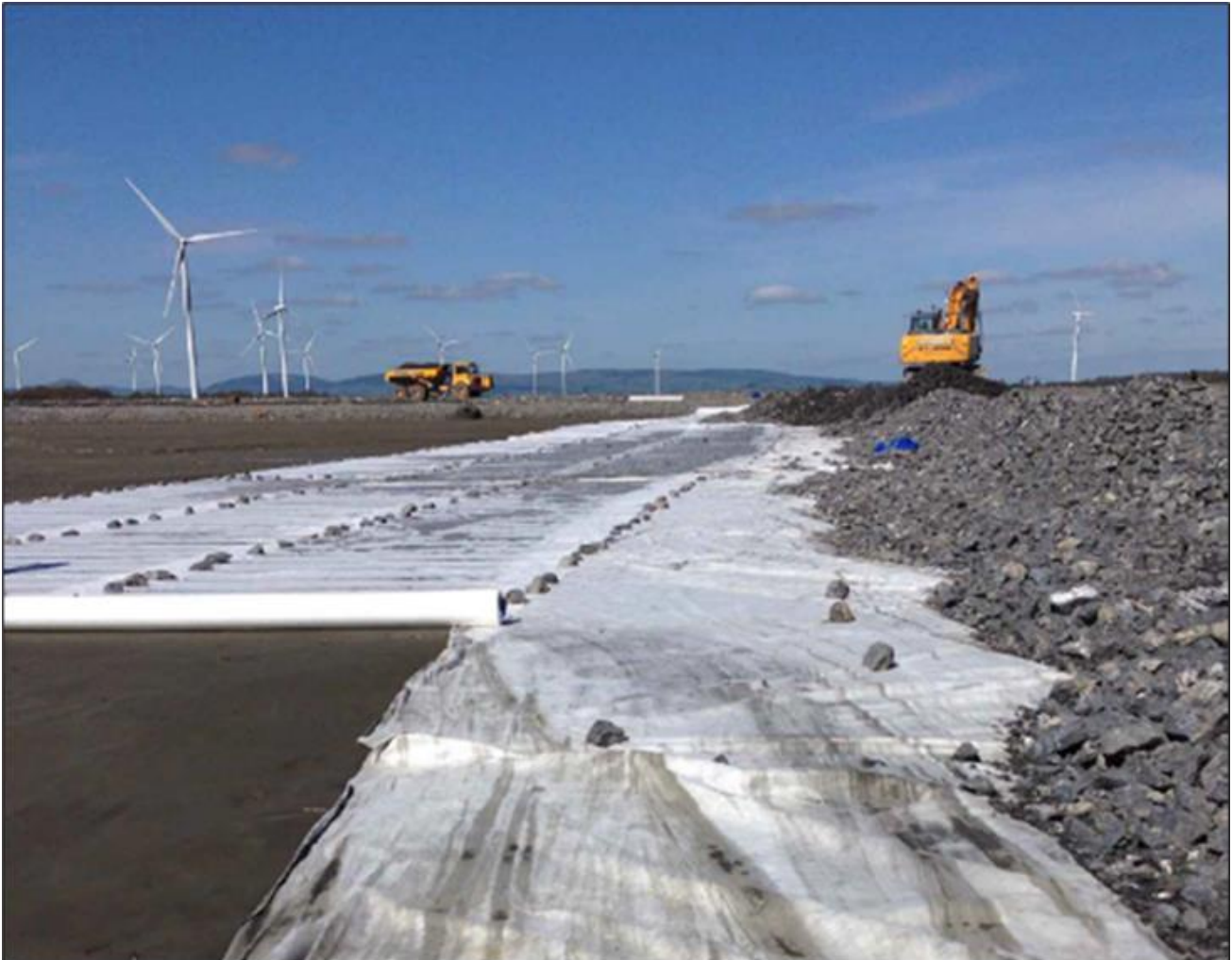
Figure 4-6: Placement of geotextile above the beached tailings
