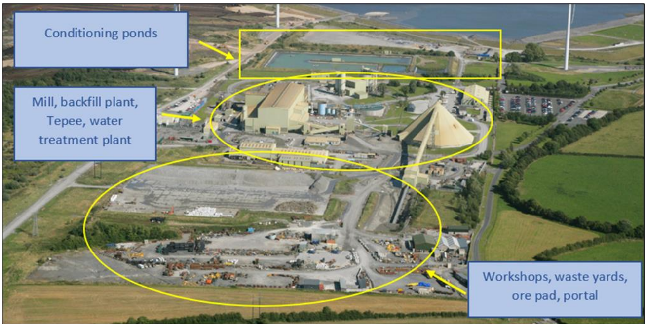
Figure 3-1: Mine Site pre demolition
