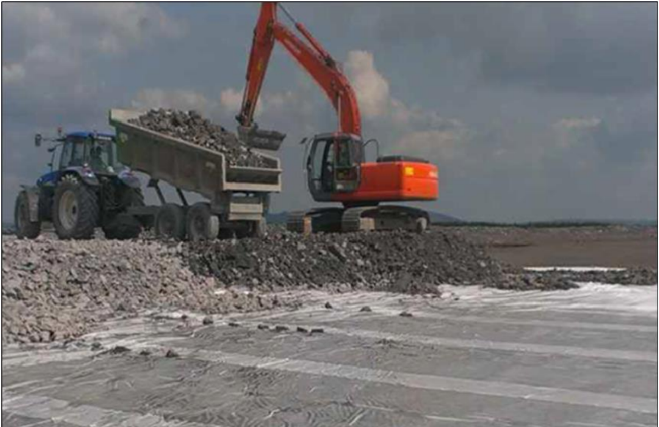
Figure 4-7: Placement of the rock cap above the geotextile layer
