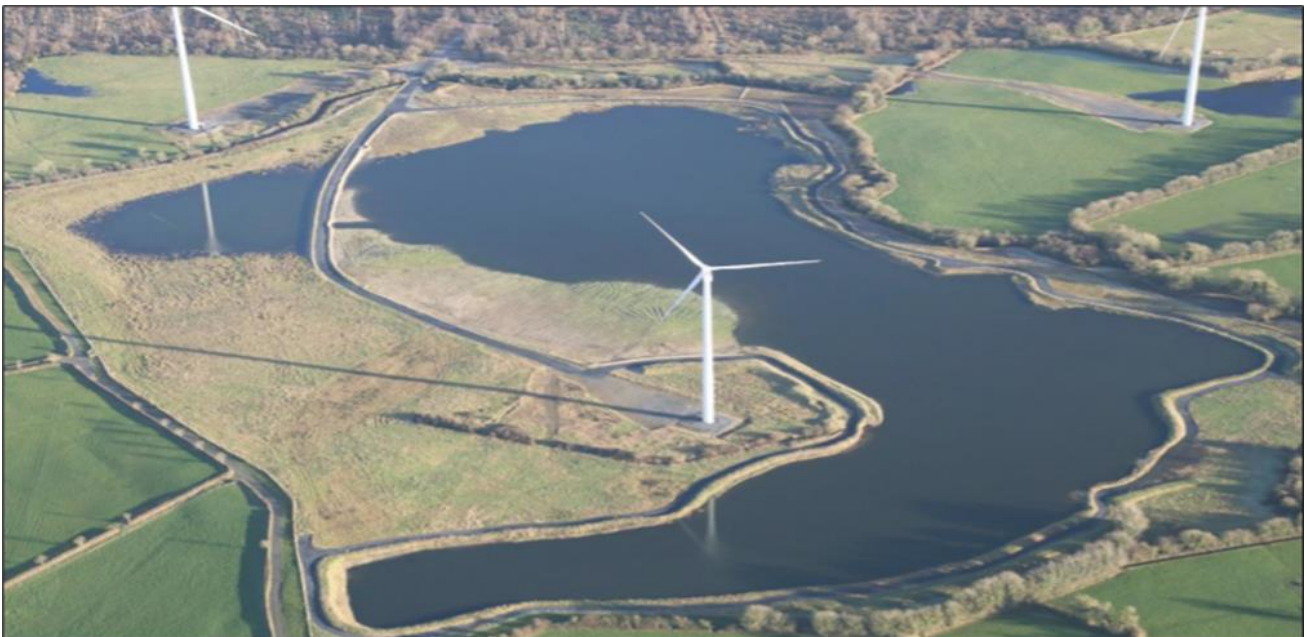
Figure 3-19: Carrick Hill post rehabilitation
