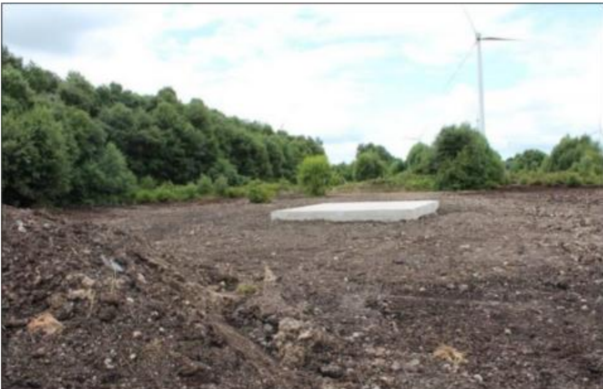
Figure 3-6: Ventilation Shaft 6 post demolition and rehabilitation
