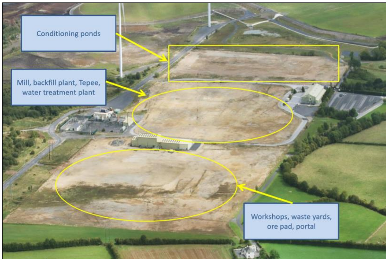
Figure 3-2: Mine Site post demolition and rehabilitation
