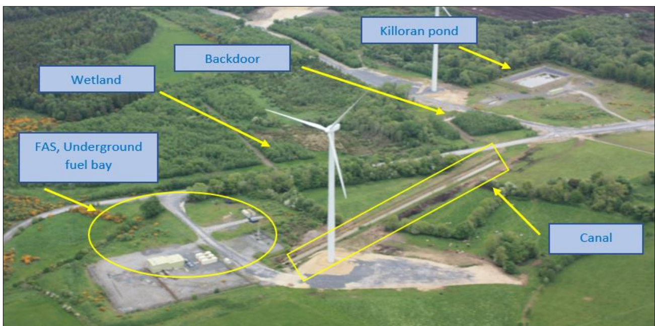
Figure 3-16: Killoran pond, canal and wetland area pre demolition
