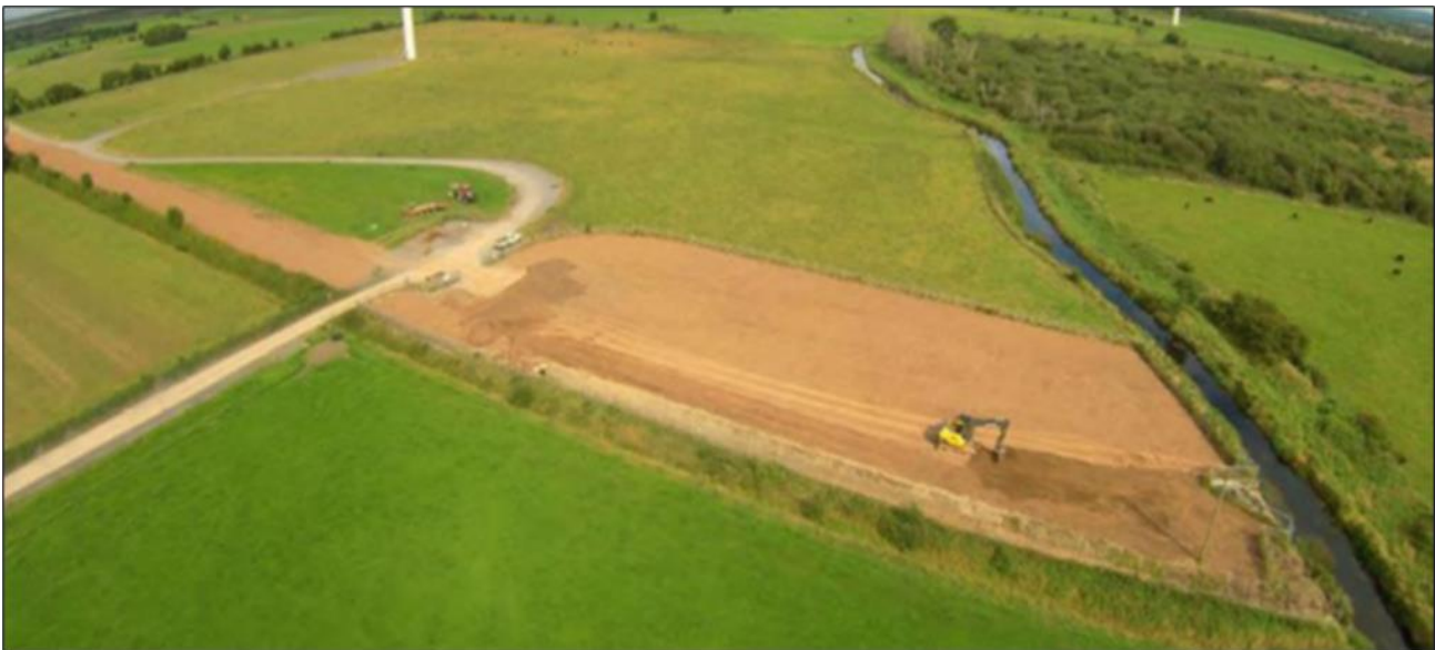
Figure 3-13: Drish Channel and Pond post demolition and rehabilitation
