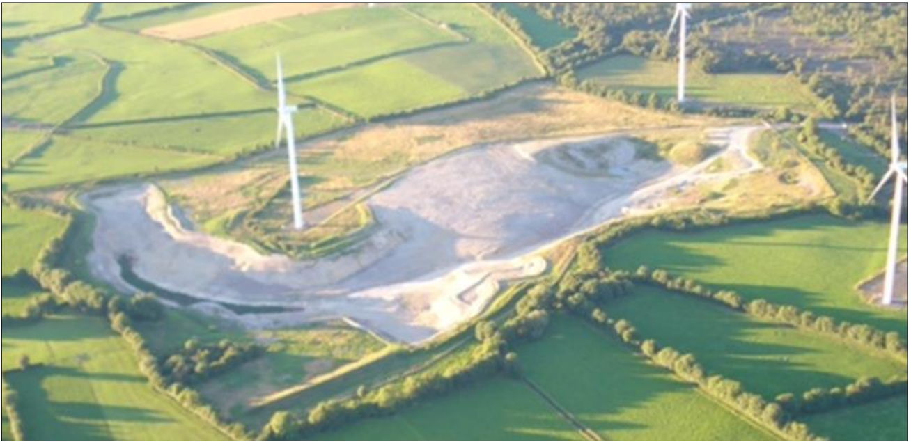
Figure 3-18: Carrick Hill pre rehabilitation
