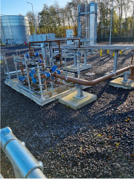
Picture 4: Fuel circulation system and bund
