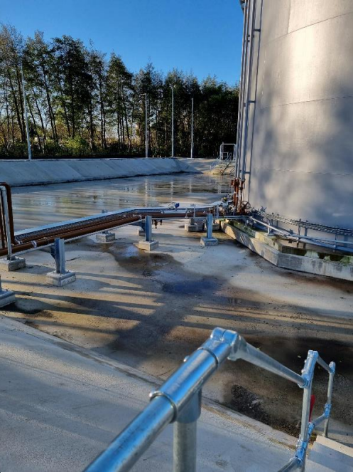
Picture 5: Fuel storage tank and bund
