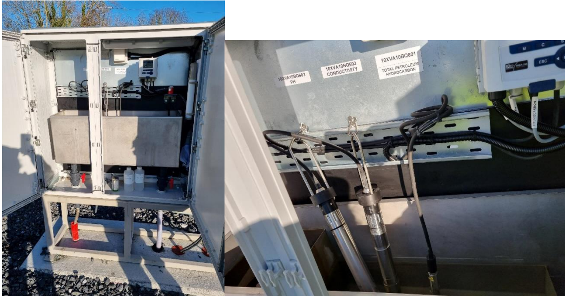
Picture 1 & 2: Stormwater Monitoring point SW1
