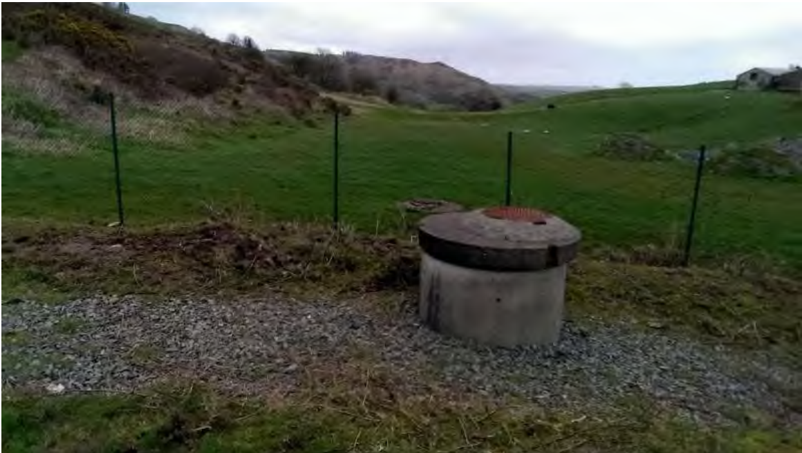
Photo 3.3 Surface water swale and discharge pipe manhole, northeast corner of landfill
