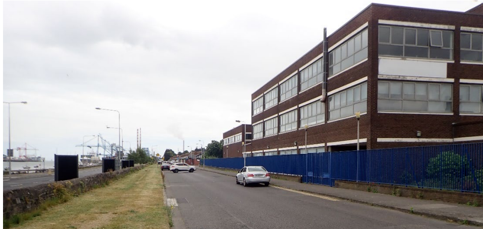
View looking east along York Road where the south-facing parapet does not survive above ground but is replaced with the curtilage fencing of Ringsend College
