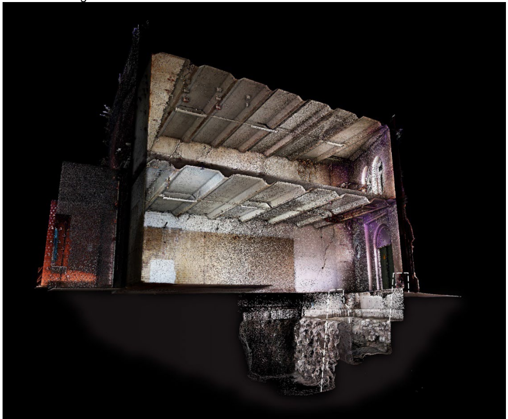
ADCO laser-scan survey showing the exposed extent of the sea wall underneath the Substation
