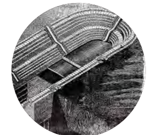
Graving Dock No.1
