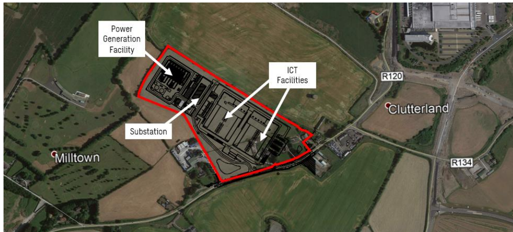
Figure 3.1: Overview of Site and DPHSL Installation
