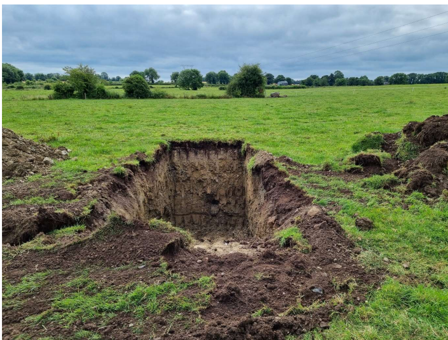
Plate 7.2 Trial pit in eastern area of the site
