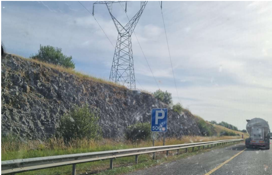
Plate 7.1 Motorway rock cutting
