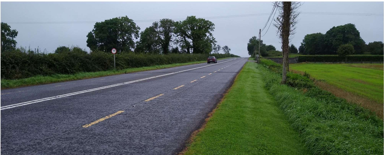
Plate 12.1 The R446 Regional Road at the Location of the Proposed Project Access Junction
