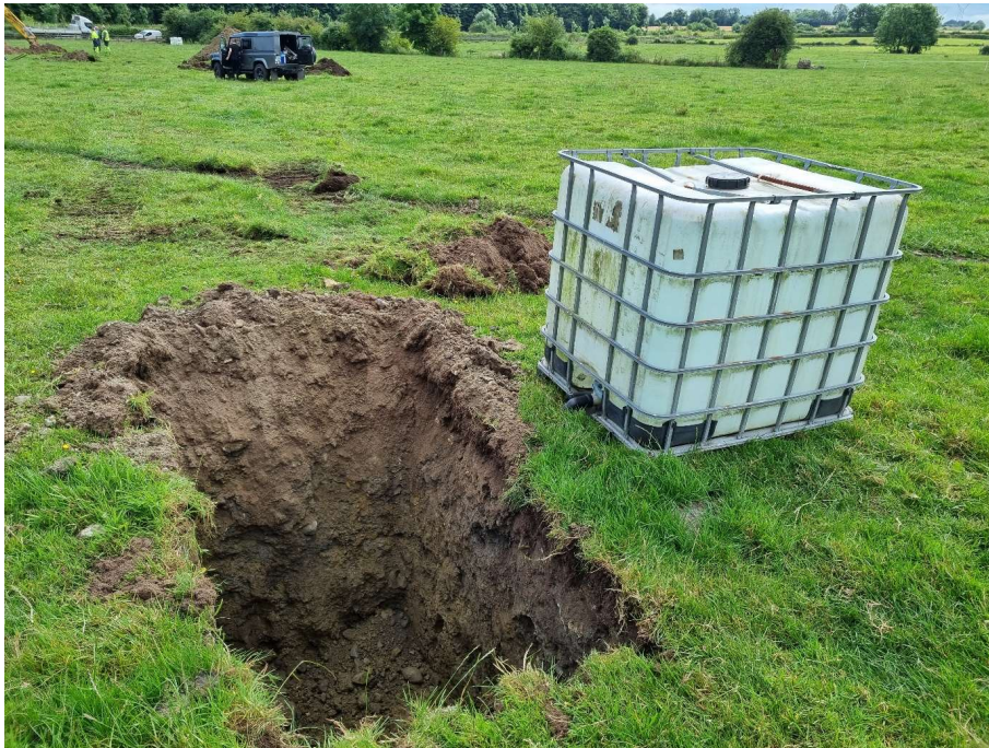
Plate 7.3 Trial pit in eastern area of the site
