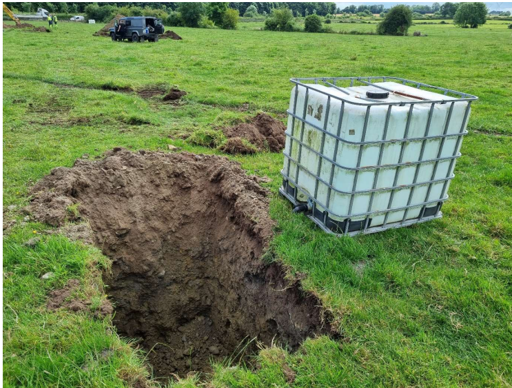
Plate 6.5 Trial Pit towards the northern area of the site
