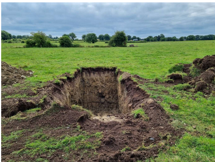
Plate 6.3 Trial pit in eastern area of the site
