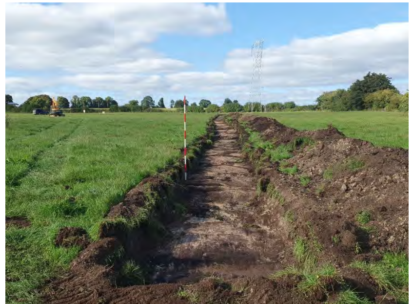
Plate 28: Trench 24, facing north
