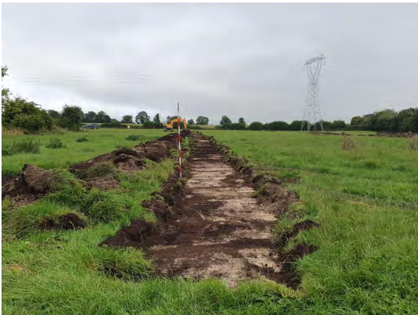
Plate 27: Trench 23, facing north
