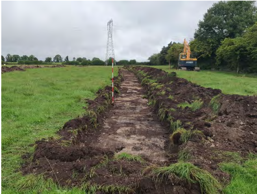
Plate 29: Trench 25, facing north
