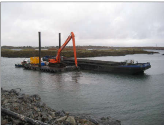
Typical Dredge Barge, Backhoe Excavator, and Hopper Barge
