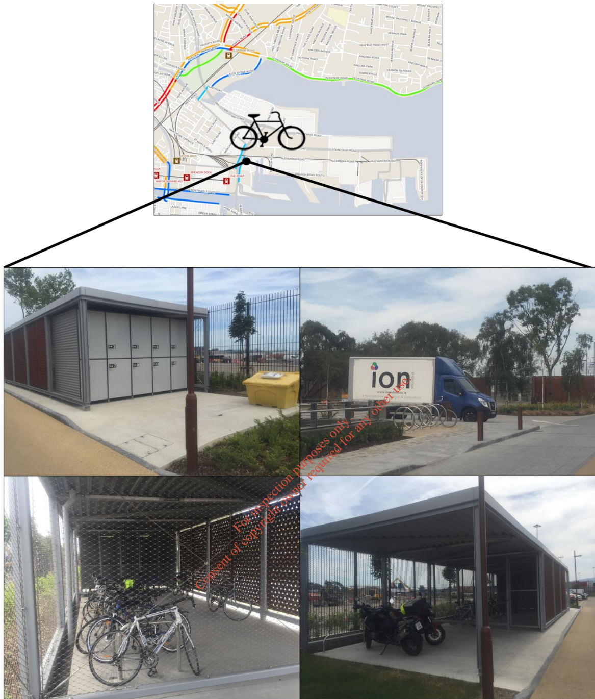
Figure 6.6 Location of Cycle Lockers at Port Centre
