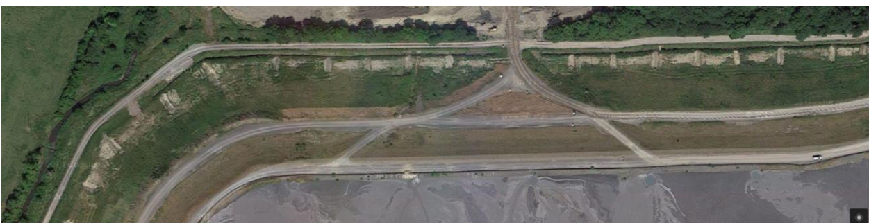
Photos showing locations of finger channels on the downstream side of the existing northern wall to be backfilled
