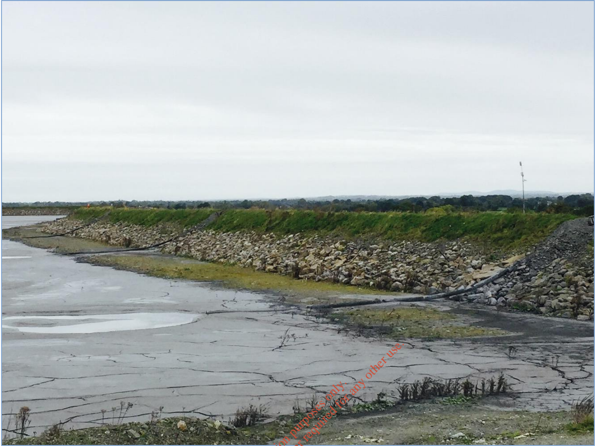
Figure 4 Typical Spigot Point
