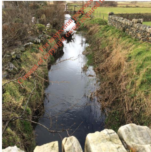
Photo 1: Ardagh 40 stream downstream of WwTP
