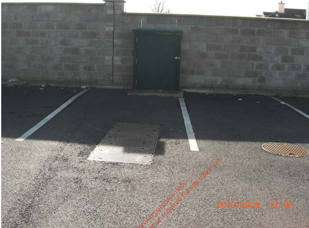
Photo KK-WWDL-207-C.1.2.1 – Pumping Station at Glen Vale
