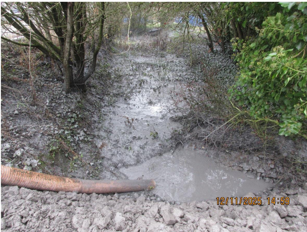
Photograph 2: Drainage ditch on near side of access road
