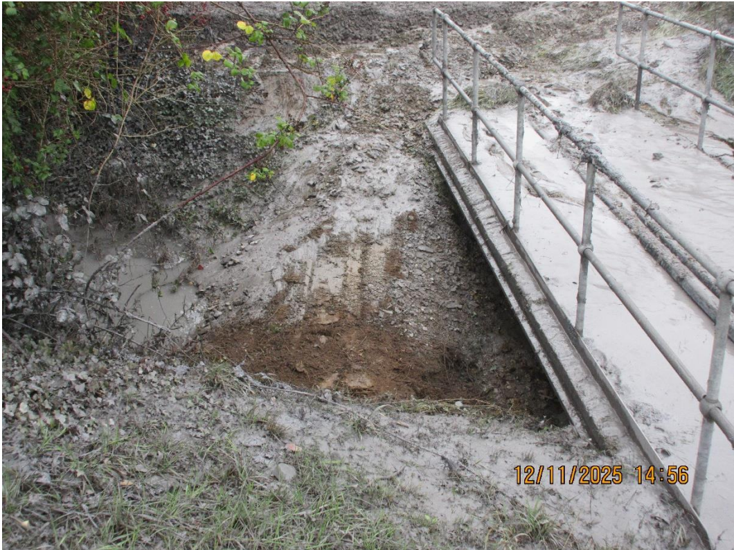
Photograph 7: Containment berm in drainage ditch
