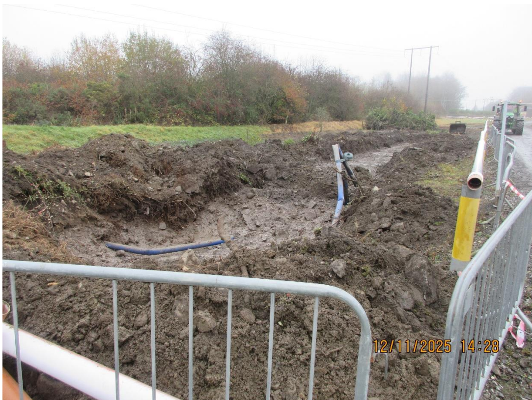
Photograph 6: Containment berm beside access road
