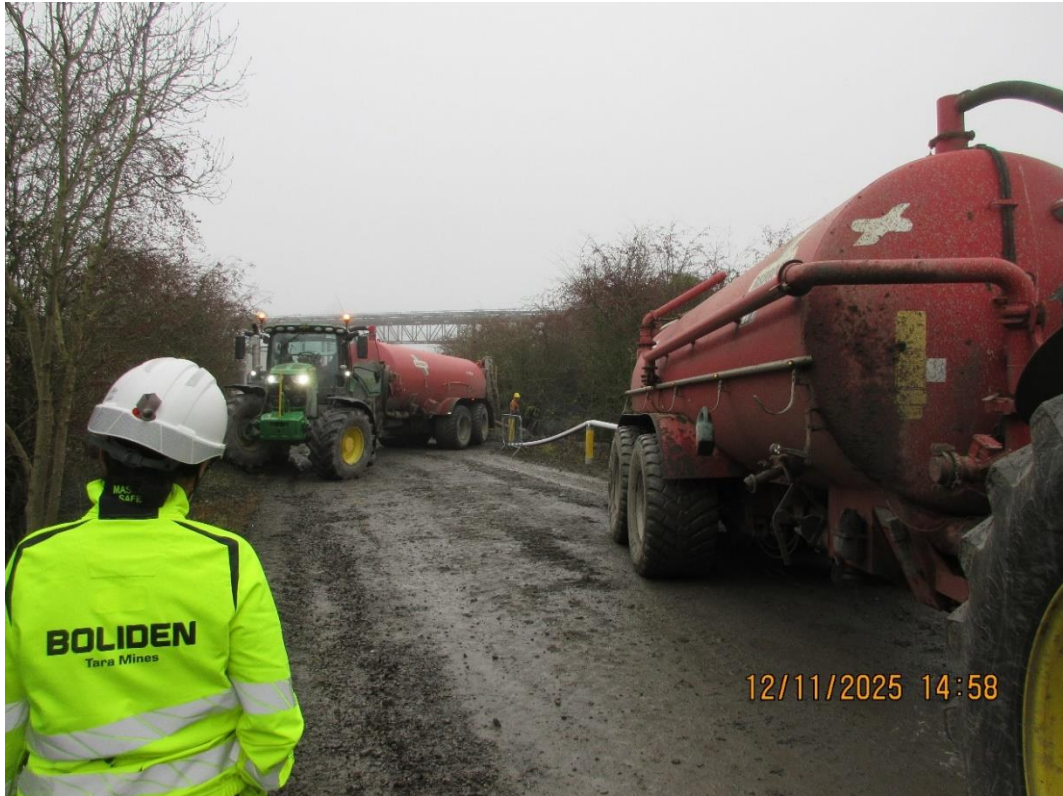
Photograph 5: Tankers extracting tailings-carrying water
